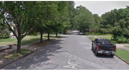
Figure 1. Especially without parked cars present, Arch Street is straight, level, and wide, which may promote speeding. 1
