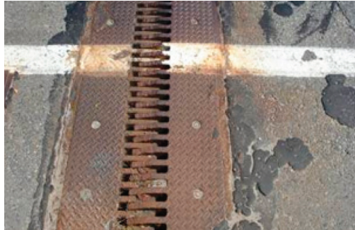
Non-Bicycle Compatible Bridge Expansion Joint
