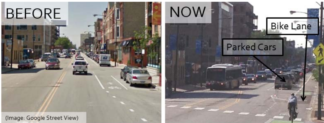
Figure 3-21. Milwaukee Ave. Chicago, IL, Before and After Installation of Protected Bike Lane
