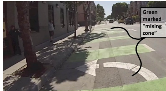
Mixing Zone with Green Coloring Photo from survey (shown): Fell St. and Broderick St. Video Location(s): Fell St. and Baker St.
