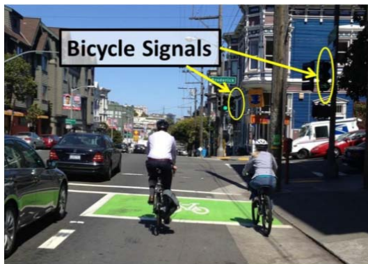
Leading Bike Interval with Bike Signal Photo from survey (shown): Oak/Broderick Video Location(s): Oak/Broderick
