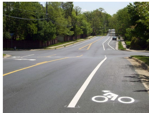
Resurfacing project incorporating Road Diets on Oak St. in Dunn Loring, VA.
