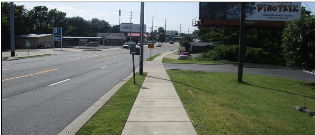
Figure 2: Bus Stop at Highway 10 and Gleneagles Lane
