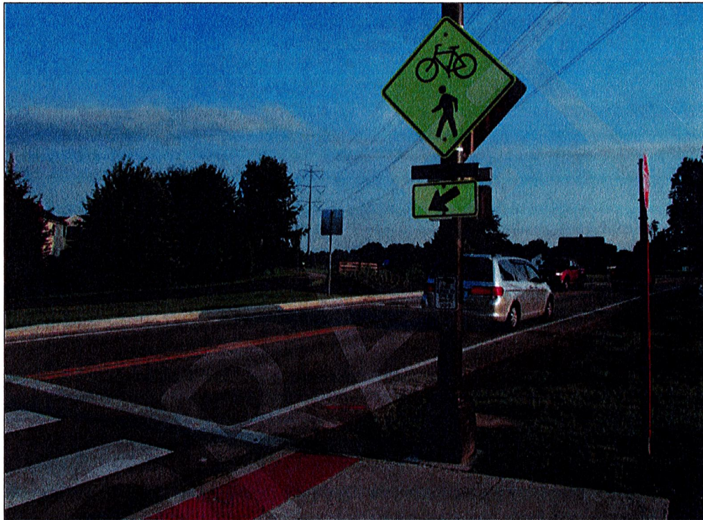
Figure 4 – Rectangular Rapid Flashing Beacon
