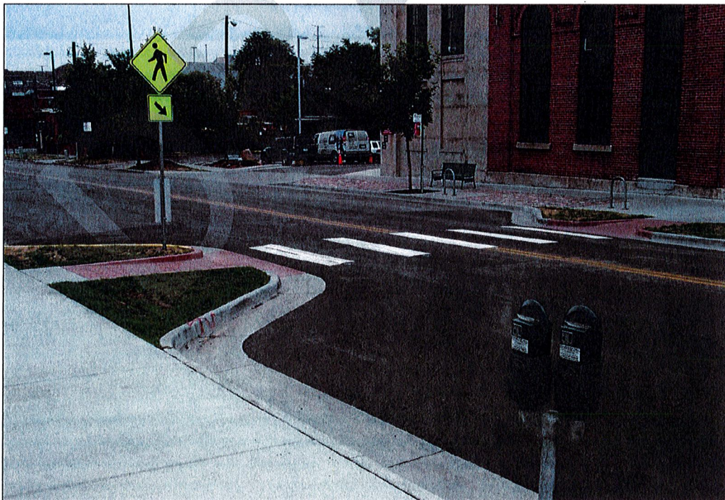
Figure 6 – Curb Extension
