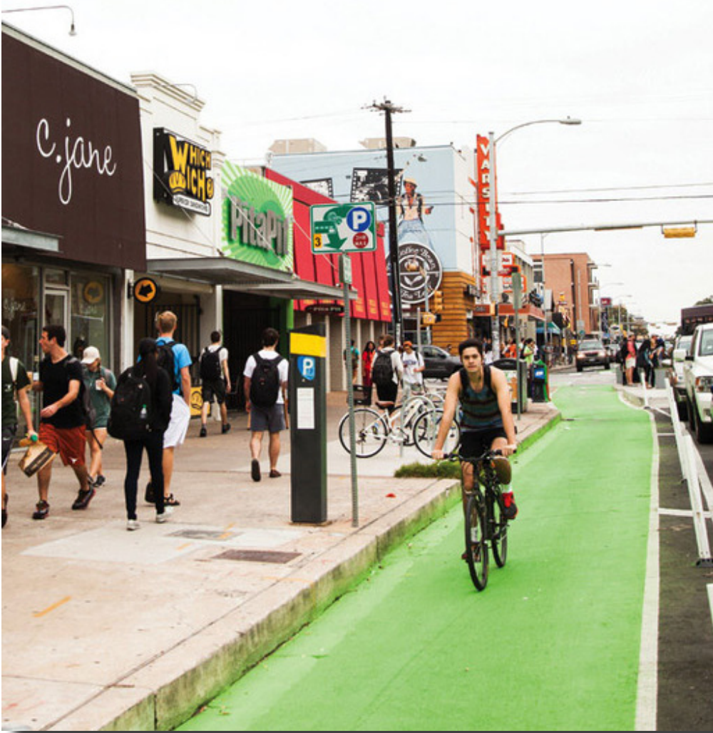
Above: Green line, or a protected bicycle lane, near the University of Texas-Austin campus on Guadalupe Street in Austin. Image credit: PeopleforBikes. Retrieved from: archinect.com/news/article/91832887/protected-bike-lanes-strengthen-city-economy-report-finds
