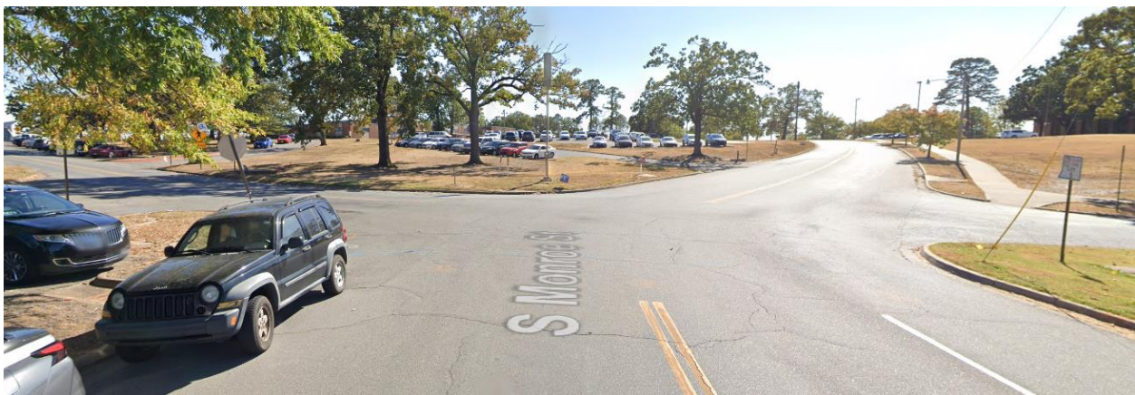
Figure 6. Crosswalk #5. An unmarked crosswalk on the north side of the Monroe and 7 th Street intersection. Crosswalk infrastructure here would increase yield compliance and physically prevent vehicles from parking illegally close to the crosswalk, like this Jeep ( Google streetview, October 2022 ).
