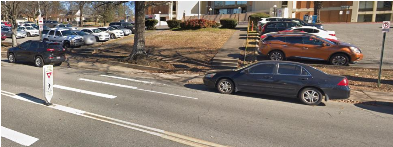
Figure 3. Crosswalk #2, east side. Parallel parking is heavily used during the workday, but not used outside of working hours. During the workday, people often illegally park too close to the crosswalk, like these two cars, creating sightline/safety issues. Getting out of the crosswalk and onto the sidewalk may be challenging for someone with a mobility device. Outside of the workday, this puts them at risk of being hit ( Google streetview, Jan. 2019 ).
