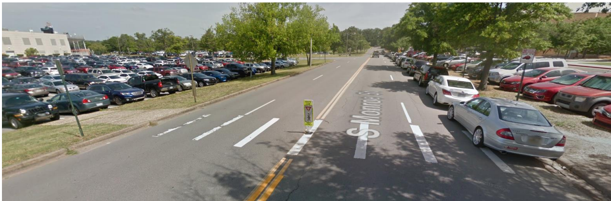
Figure 5. Crosswalk #4. No curb ramp or sidewalk on east side. No curb ramp on the west side. No break in War Memorial parking to allow access to the sidewalk. Note the car parked in the crosswalk. ( Google streetview, July 2016 ).
