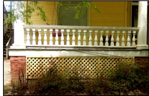
Figure 60. This front porch on 15 th Street has many of the design features found throughout the district: brick piers, lattice work between the piers, and well-proportioned posts, hand railing and balustrade.
