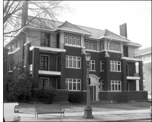
Fig. 146. Rainwater Apartments. 519 E. Capitol
