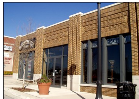
Figure 79. This new building uses pilasters to break up the massing of its façade.
