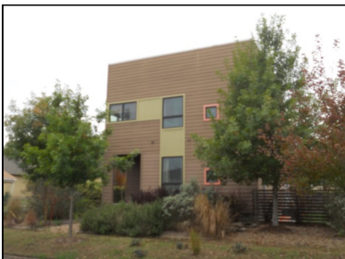
Figure 68. 324 E 15th Street
