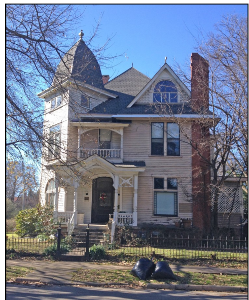
Figure 119. Chisum House, 1320 Cumberland Street
