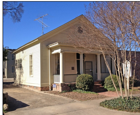
Figure 129. Reigler Cottage, 610 Rock Street
