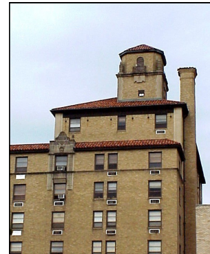
Figure 139. Albert Pike Hotel, 701 Scott Street
