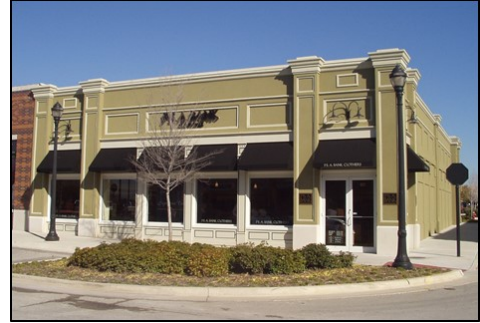
Figure 78. This new infill commercial building has many of the characteristics consistent with these design guidelines, including: front setback on the street ROW, a flat roof screened with a parapet wall, the use of pilasters to break up the façade into vertical bays, paneled wood bulkheads, transoms, awnings, and a well-defined primary entrance off the associated street.
