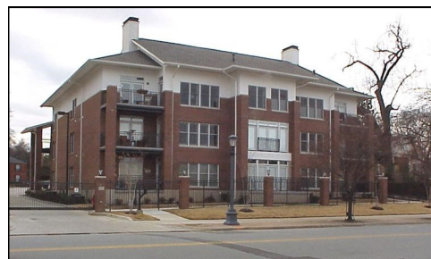
Figure 71. 515 E Capitol Avenue
