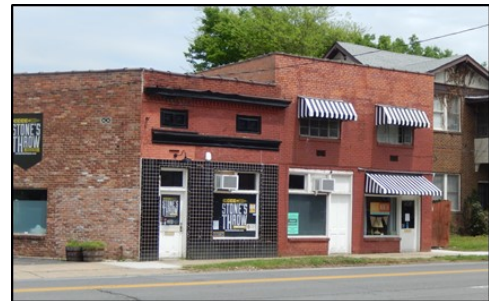
Figure 76. Regardless of the alterations that have occurred to these buildings on E. 9 th Street, a new commercial or mixed-use building near them having more than three (3) stories may be out of scale with this node's historic context.
