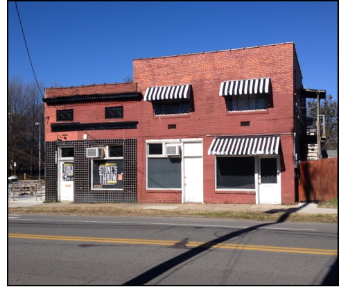
Figure 38. Commercial node on 9th Street
