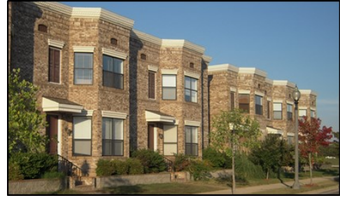
Figure 58. These new townhouses have utilized corniced parapet walls to visually screen their flat roofs.
