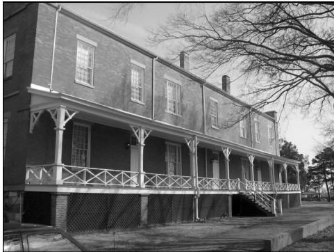
Figure 107 The Arsenal Building (south elevation)
