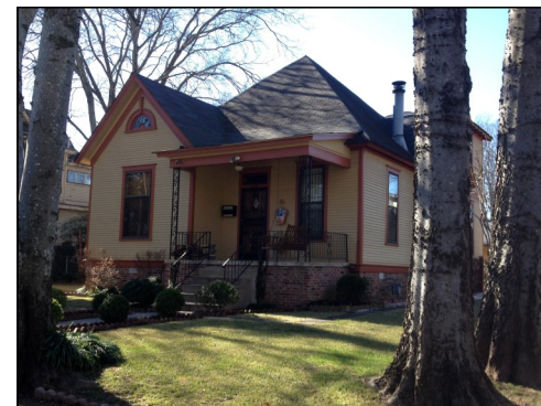
Figure 130. Hanggi House, 1314 Cumberland Street
