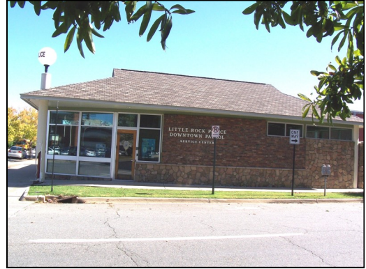
Figure 83. 301 E Capitol Avenue
