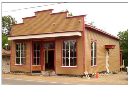
Figure 81. Clapboard siding would be an acceptable cladding for a new commercial building in the district. However, since brick is the more dominant cladding for this building type, brick should continue to be the primary material for most new commercial and mixed-use buildings in MacArthur Park.
