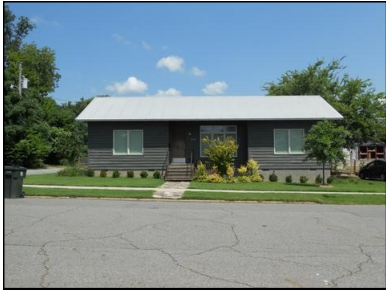
Figure 62. 320 E 15th Street
