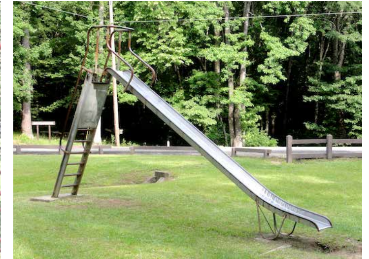
In addition to having unacceptable surfacing under it, this metal slide may become superheated on excessively hot days.
