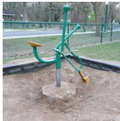
The exposed footer on this equipment is a hazard and should be covered with surfacing.
