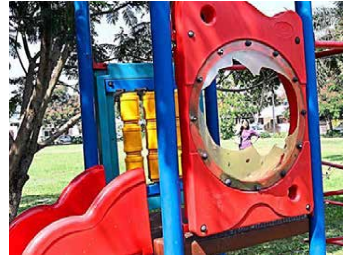
This vandalized bubble panel has been damaged and should be replaced.
