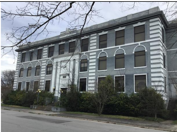
Joshua Building at 2501 State Street. This building was the Little Rock College 1908-1916, St John's Seminary 1911-1916 and 1920-1930, St Joseph's Orphanage 1916-1920, the Catholic Boys School in 1930-1961. EOA was here in the late 1990s.
