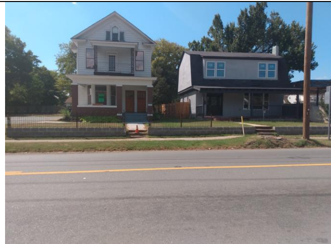
2510 S Arch Street (left) has been renovated by owner Deryan Coleman and a new parking lot installed. 2008 Arch (right) has been recently renovated.
