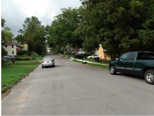
New sidewalks at 28 th and Marshall Streets.
