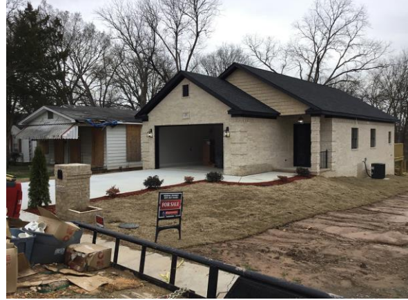
3023 S Main was under construction.
