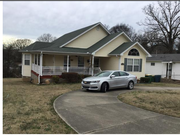
3104 Gaines Street shows new construction.
