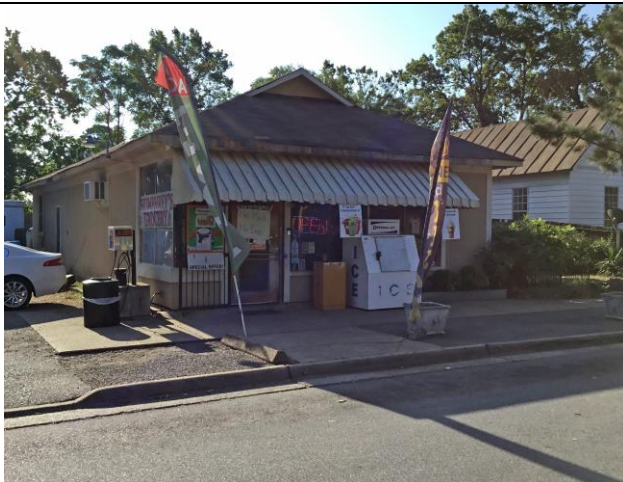
The Humphrey Store at 2901 S Wolfe Street.
