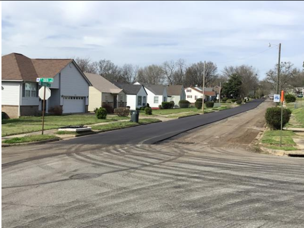
Cross Street from Roosevelt south in process of being repaved.
