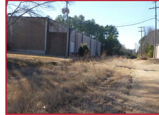
Railroad corridor in south Little Rock.
