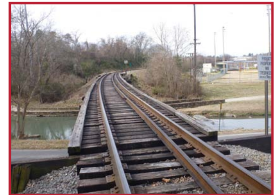
Active rail corridor over the Hot Springs Creek Greenway.
