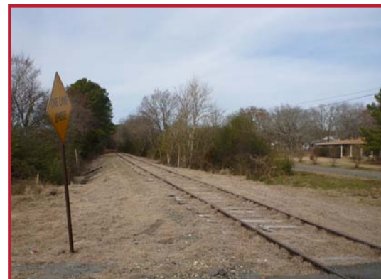
Railroad corridor in Hot Springs.
