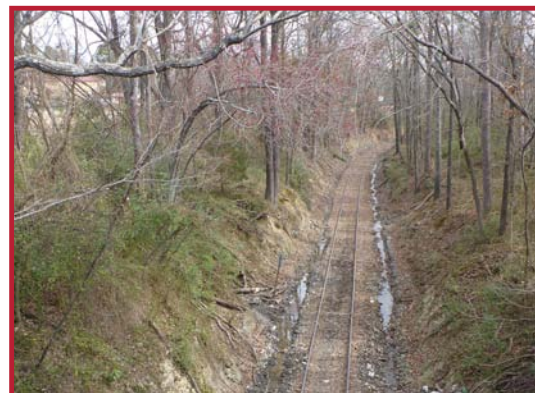
Railroad corridor in Hot Springs.
