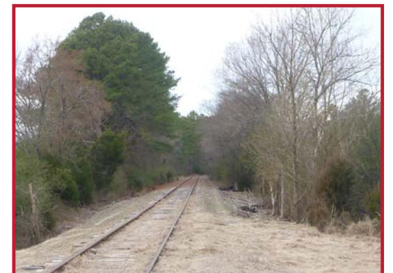
Railroad corridor in Hot Springs.
