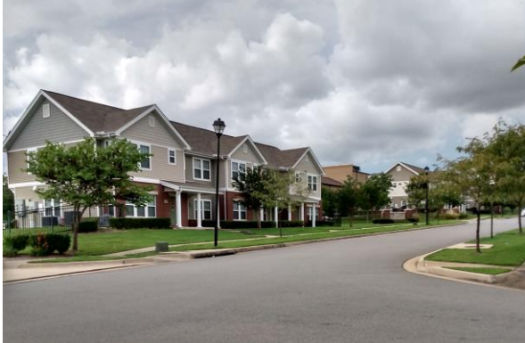
Tuxedo Court renovations.
