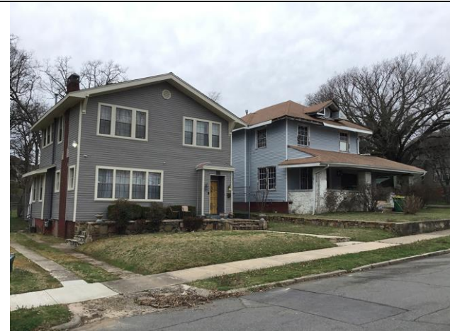
2904 Gaines on left has been recently renovated.
