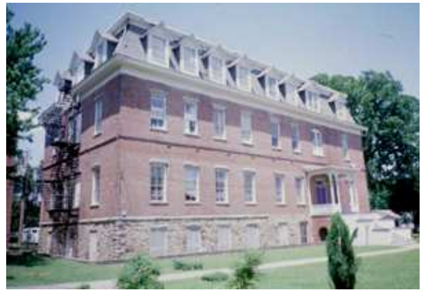
Main Building, Arkansas Baptist College 1600 South Doctor Martin Luther King, Junior Drive 1893 school for black theologians Listed on 4/30/1976
