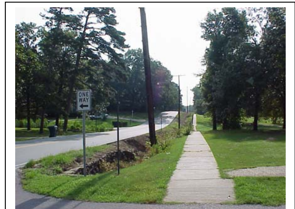
Open Drainage Ditches on W. 32nd Street
