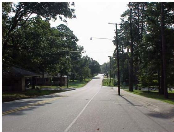
Lack of Sidewalks around Elem. School
